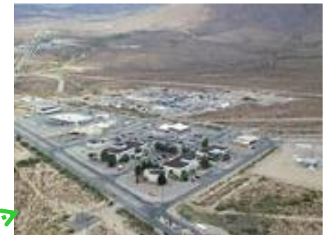
White Sands Ground Terminal, NM
