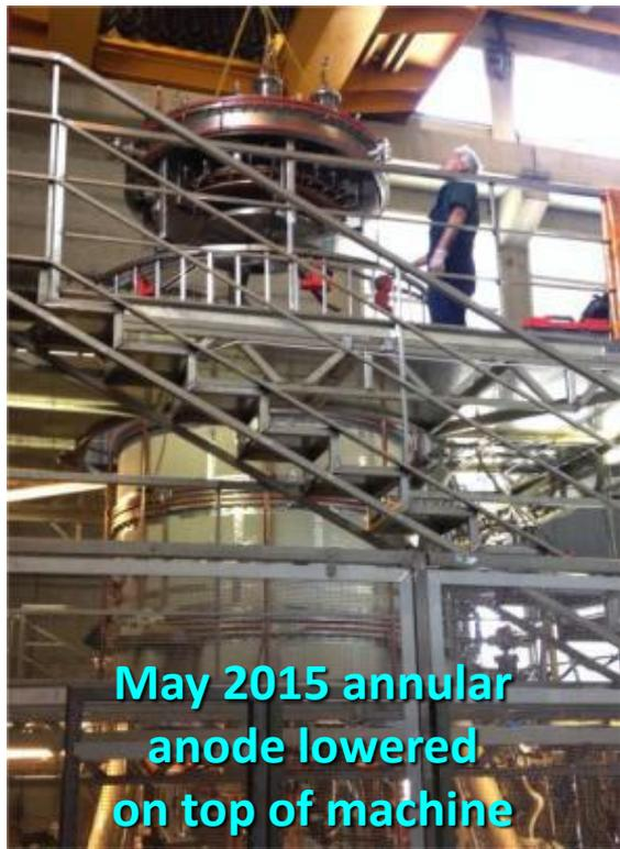
May 2015 annular anode lowered on top of machine
